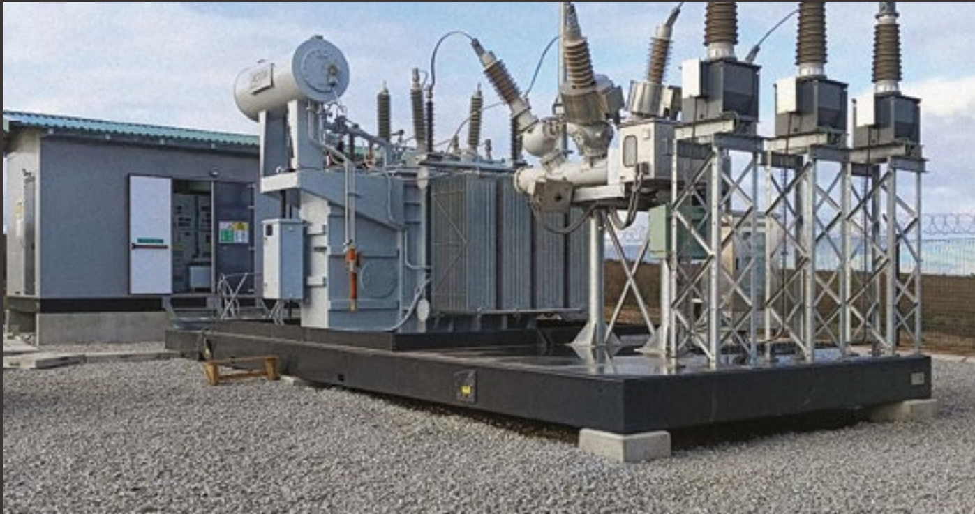
Heavy-duty 16m x 5m galvanised steel skid platform with banded grating and C5M marine-grade coating for corrosion resistance. Includes a 4,000 L polyurethane-lined integrated sump for secure high-voltage infrastructure containment.
